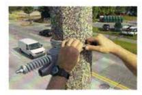
Mount top and bottom of bracket to pole with metal bands. Secure metal bands with screw driver.
