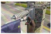
Install fiberglass arm and insert pin into nose and arm.
