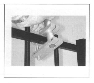
Insert threaded rod into bottom section of rail mount. Make sure that rail is between the two rail mounts and between flagpole and threaded rod.
